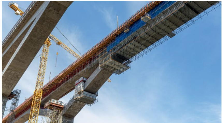
The 85 m high and 485 m long Filstal Bridge brings together all the challenges of bridge construction – a sophisticated construction method with slender superstructures and high bridge piers that widen in a Y-shape at the crown, high architectural concrete requirements and a narrow time window to meet the completion deadline.
