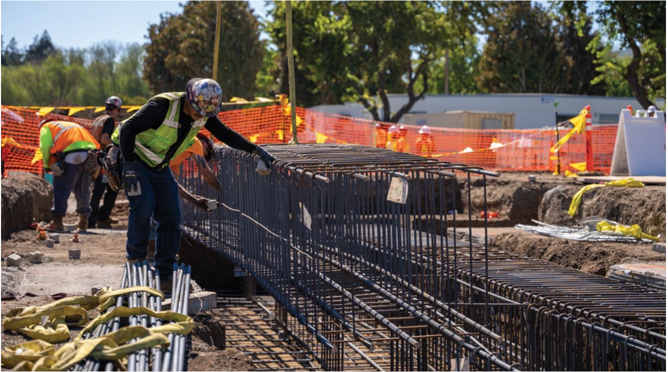
The installation of rebar cages. Projects can be delivered faster and safer, through the application of prefabrication and VDC, and the utilisation of design resources and strategic partnerships.
