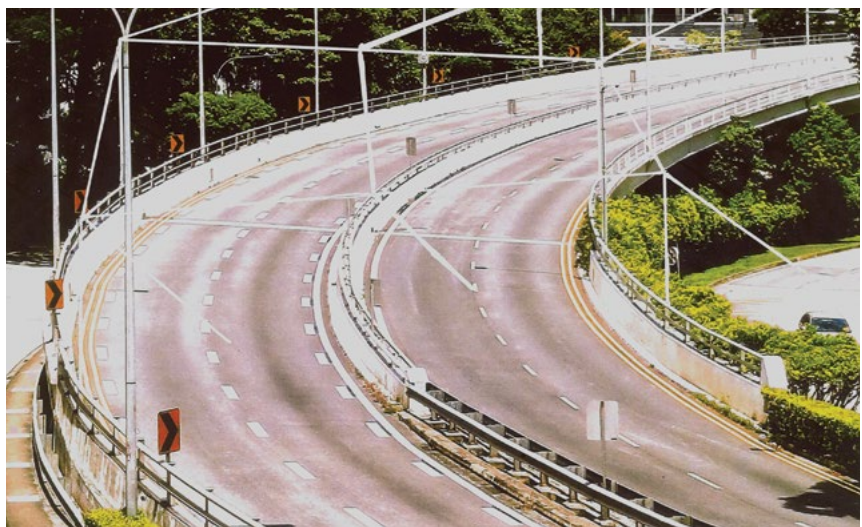
Figure 2: Flyover solar highway.
