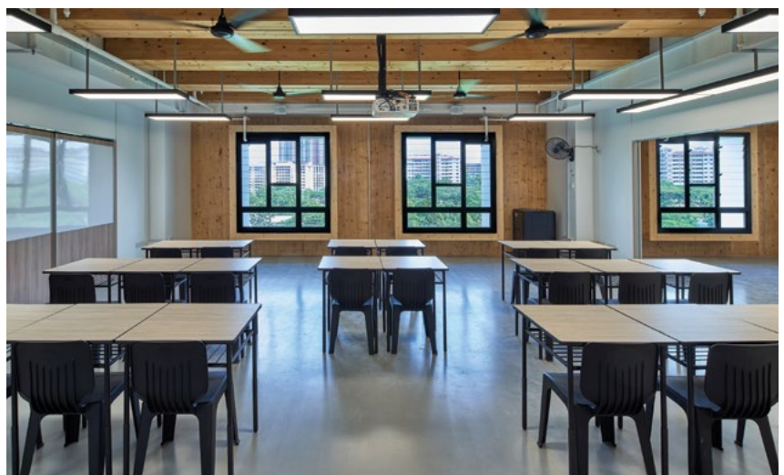
The interior of a classroom. Using Mass Engineered Timber improved buildability and contributes to environmental sustainability.
