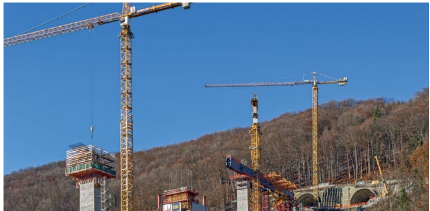
The slender reinforced concrete shafts sprouted upwards, cycle by cycle, with the aid of the rail-guided RCS climbing formwork.
