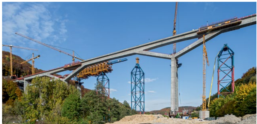
The cantilevered parapets on the west bridge were constructed in 24 m sections using a total of four VARIOKIT Cantilevered Parapet Carriages.
