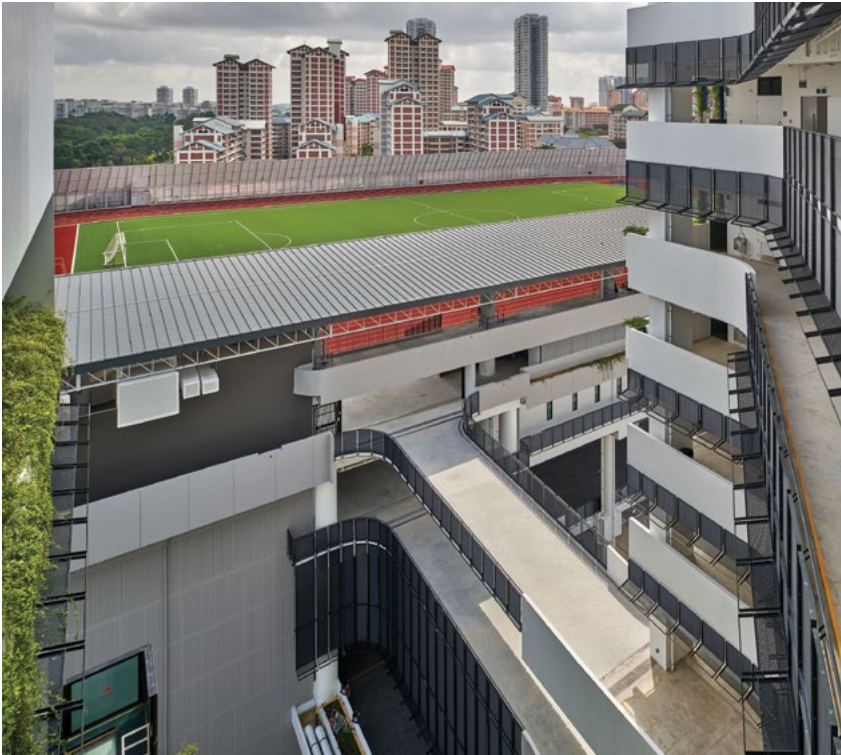
The elevated running track and field.
