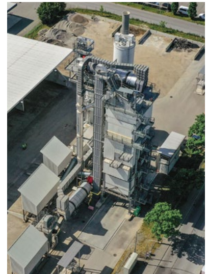
The Ammann ABP HRT asphalt-mixing plant.
