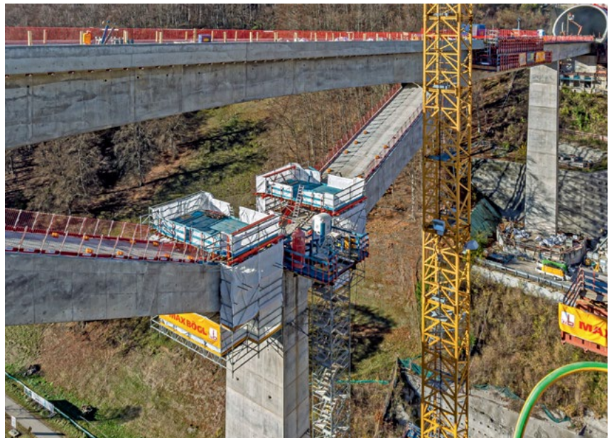
PERI engineers designed a rail-guided finishing carriage, by combining the PERI UP Scaffolding System with VARIOKIT and RCS climbing technology in order to work on the inclined piers.
