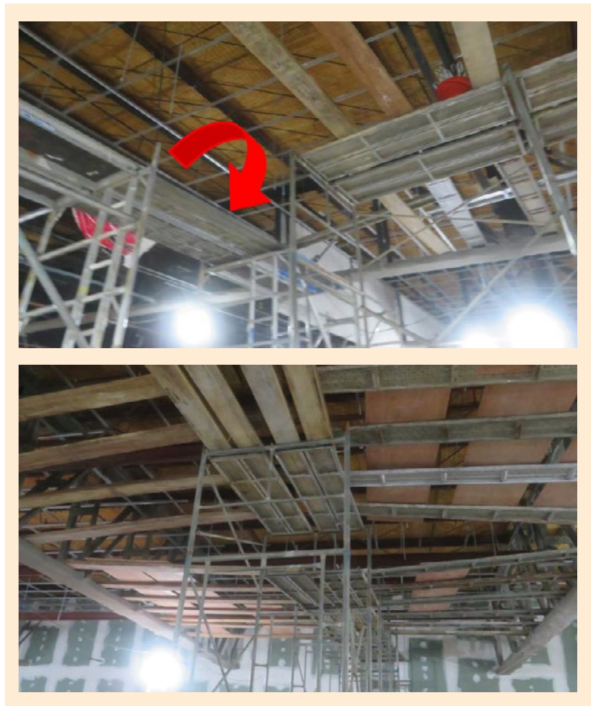
MOM issued Stop-Work Orders (SWO) to worksites in the Construction industry with unsafe conditions and practices that posed imminent danger to the workers. Image (on top): At another site, toe-boards and guardrails were not provided on the sides of the work platform at a height of more than 2 m, from where workers could fall. Image (below): Workers were found working on work platforms that were not closely boarded and properly secured, which may lead to accidental displacement (i.e. shifting of the platform).
